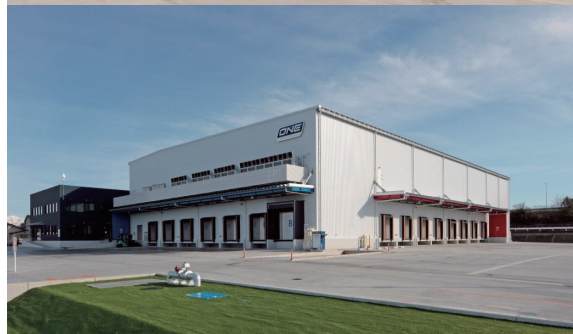
Toyama West TC (Frozen & Refrigerated Warehouse) [Toyama]
