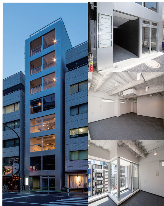
Toranomon SE Building [Tokyo]
